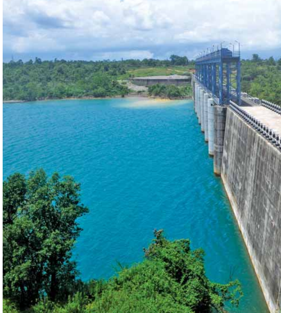
(Above and right) The Kopili Hydro Electric Project, Assam.
