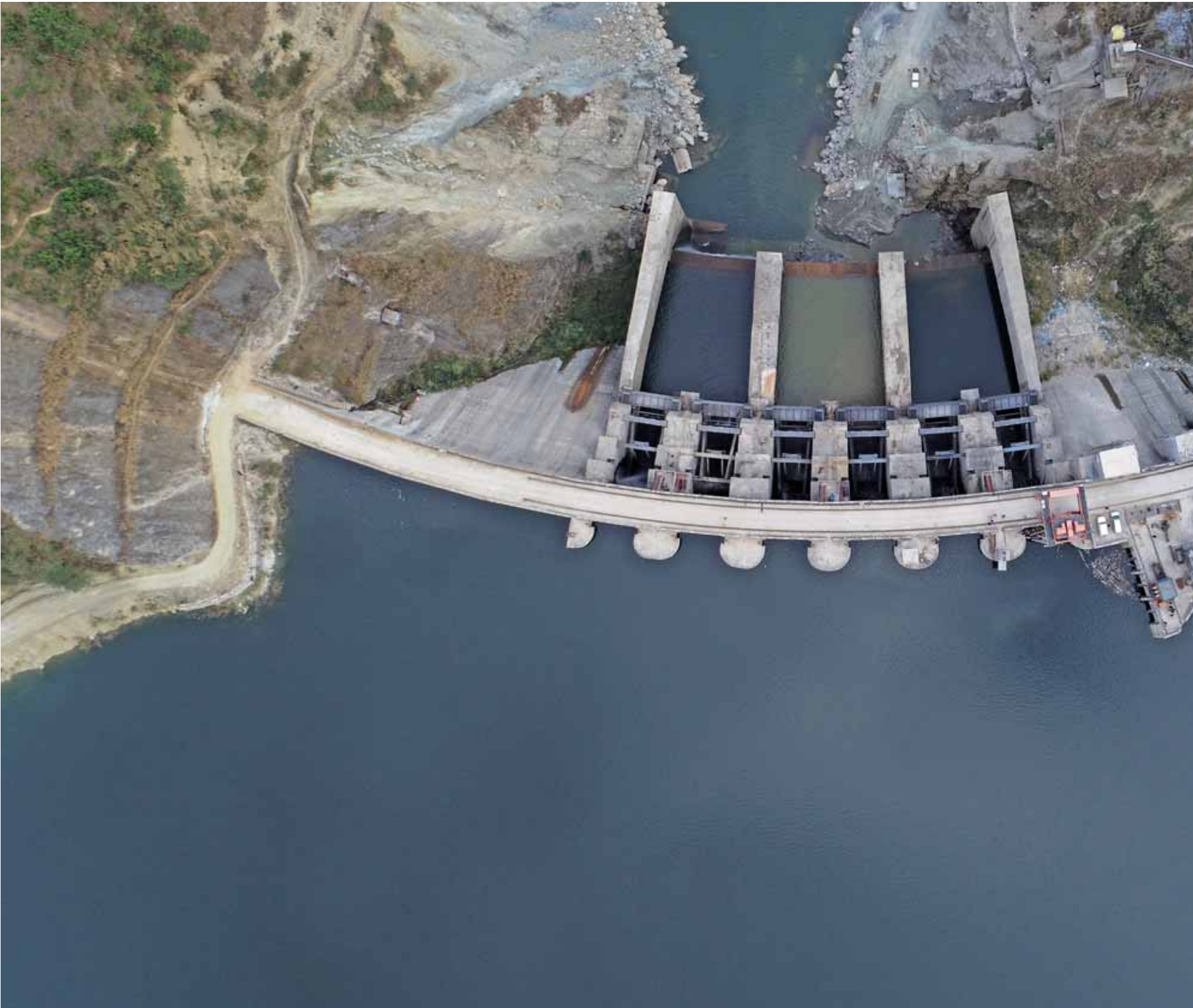
The Kameng Hydro Power Station, Arunachal Pradesh.
