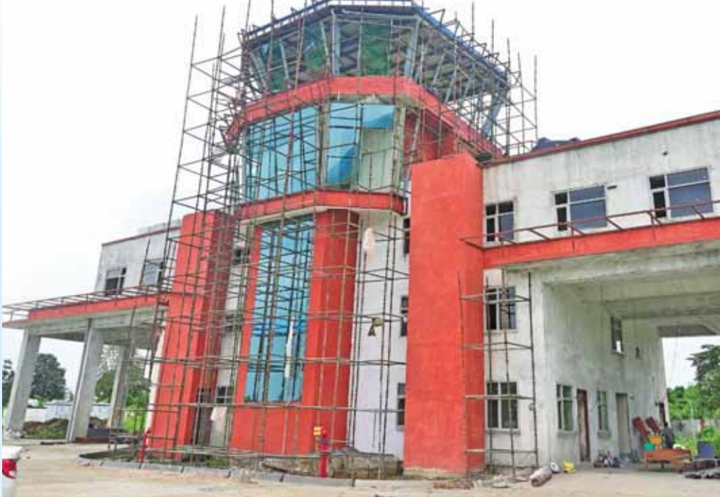
(Above) Construction of New Air Traffic Control Tower, Tezu Airport, Arunachal Pradesh; (Below) Shillong Airport, Meghalaya
