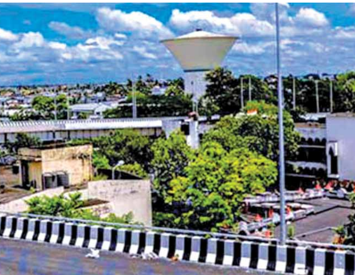
Flyover road in the state's capital town of Agartala, Tripura.
